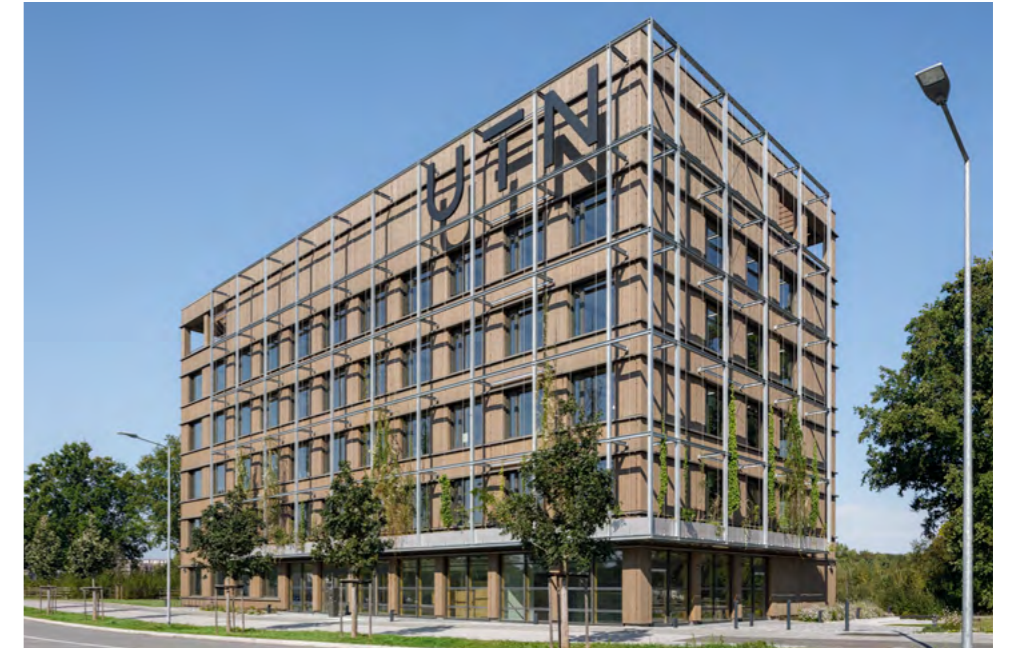
Focus on sustainability and modern construction methods Cube One © Stefan Meyer
